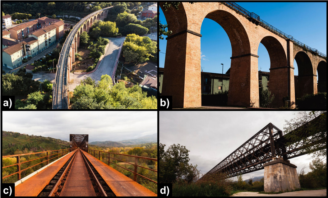
Figure 20 - a) and b) views of the Milano Bridge, c) and d) views of the Ponte Principe.
