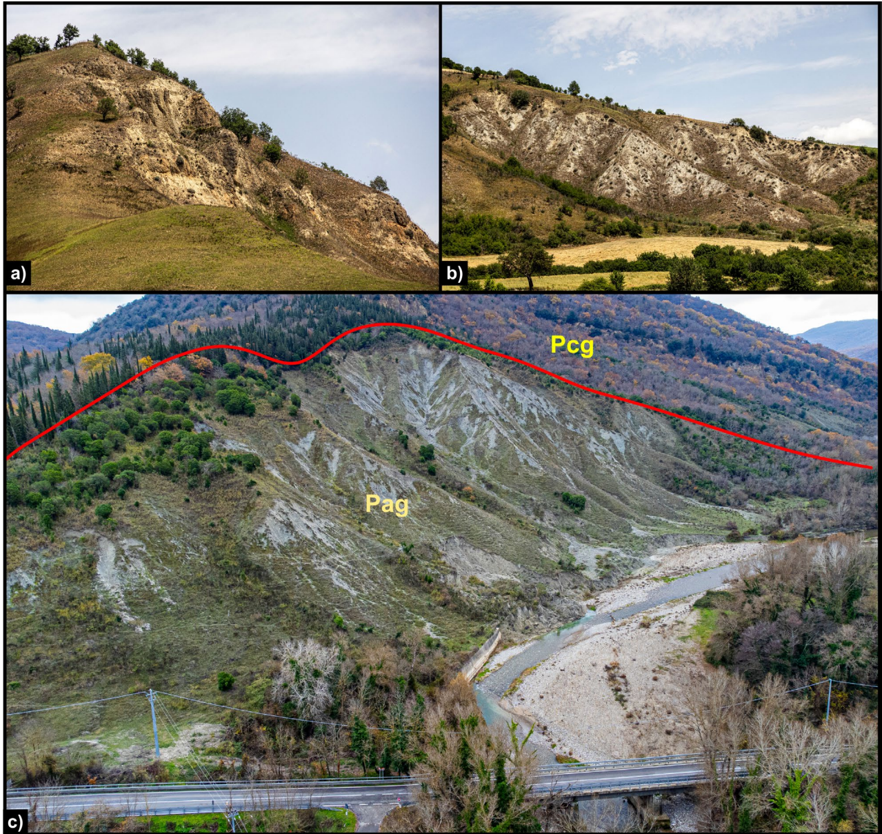
Figure 77 - Various types of slope instability affecting LU 5: a) Collapse in Pliocene sands, b–c) Badland erosion at the confluence of the Atella fiumara with the Ofanto River. The red line marks the contact between Pliocene clays (below) and Pliocene conglomerates (above), also highlighted by the vegetation change.
