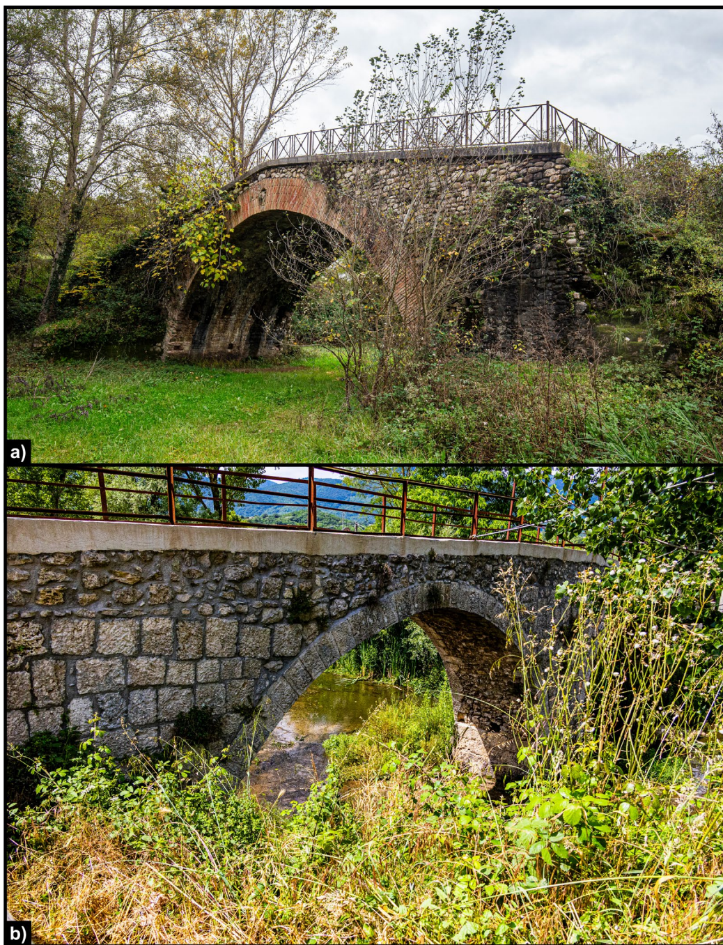
Figure 88 - a) Hannibal's Bridge at Spineto (San Mango sul Calore) along the Calore River, b) Roman Bridge along the Ofanto River at Alifano (Lioni).
