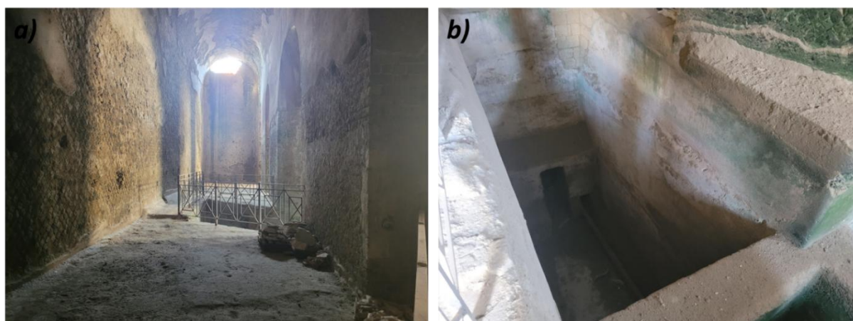
Figure 9.7. (a) Cento Camerelle reservoir, internal view; (b) Underground reservoir in Cento Camerelle (photo by Michele Ginolfi).
