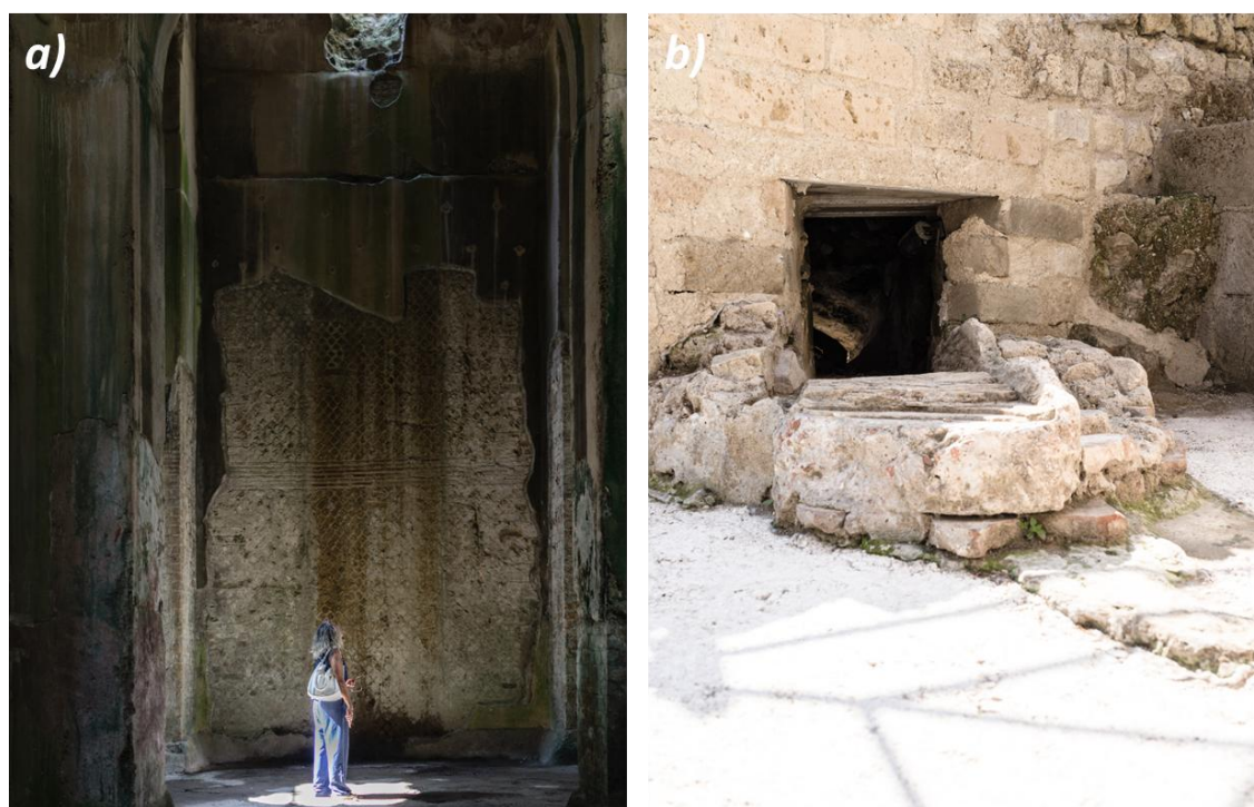
Figure 9.6. (a) Internal view of Piscina Mirabilis reservoir, on the wall is still visible cocciopesto ; (b) conduit conveying water in reservoir; several conduits were present, some of them actually are not still visible (photo by Giovanni Minervini (a) and Libera Esposito (b)).
