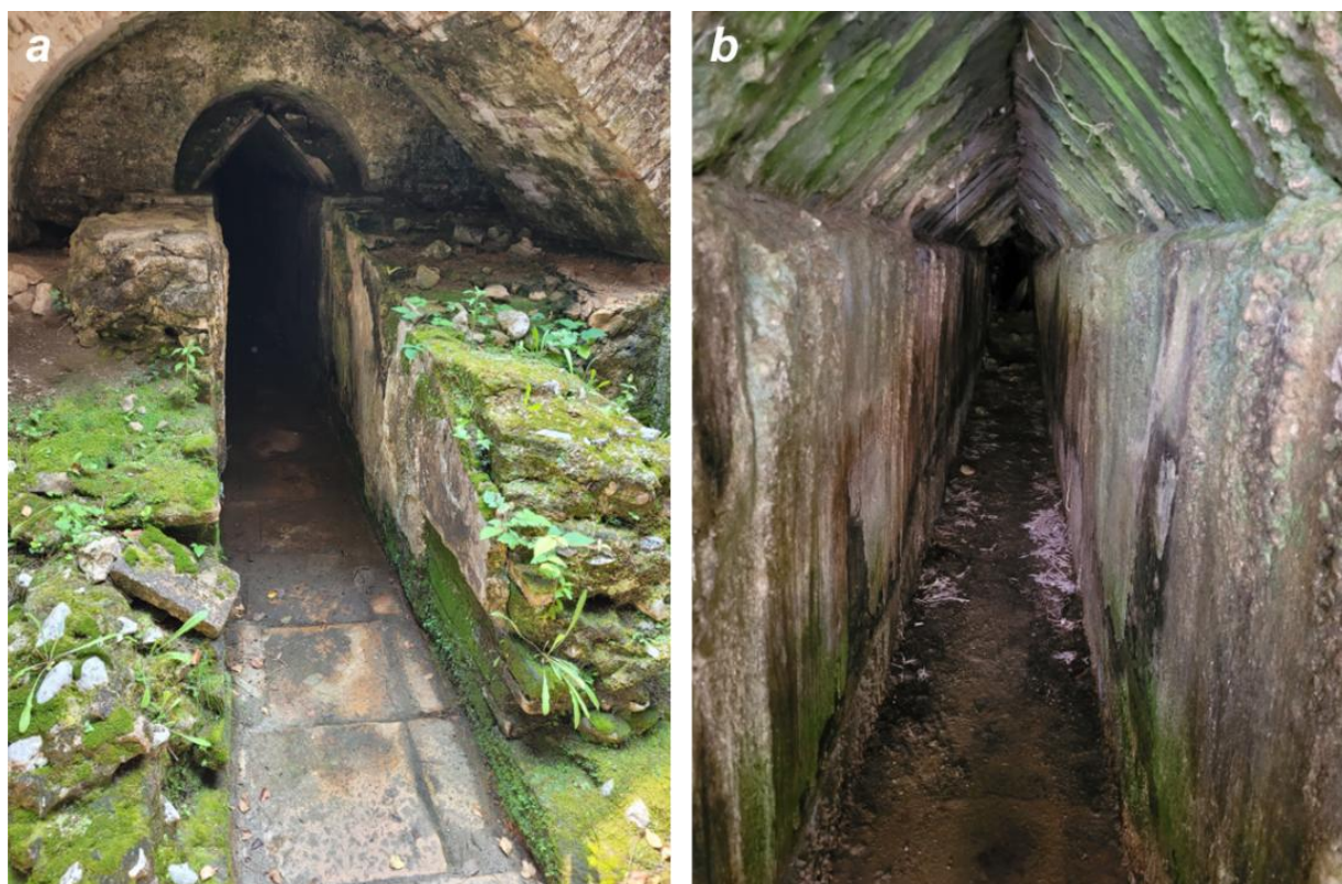
Figure 9.8. Remains of Sannitico Aqueduct (a) entering and (b) detail of the internal channel (photo by Libera Esposito).
